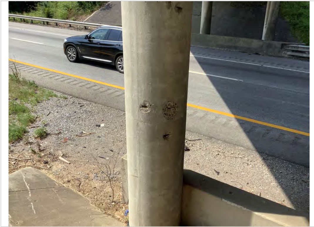
Typical spall on bents
