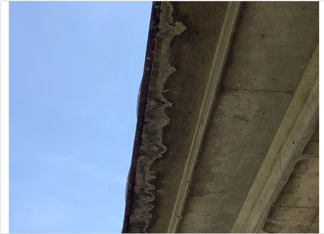
Typical delaminated areas in overhang
