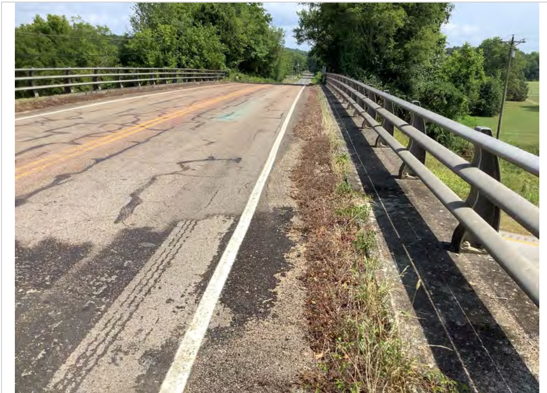
Debris on top of deck
