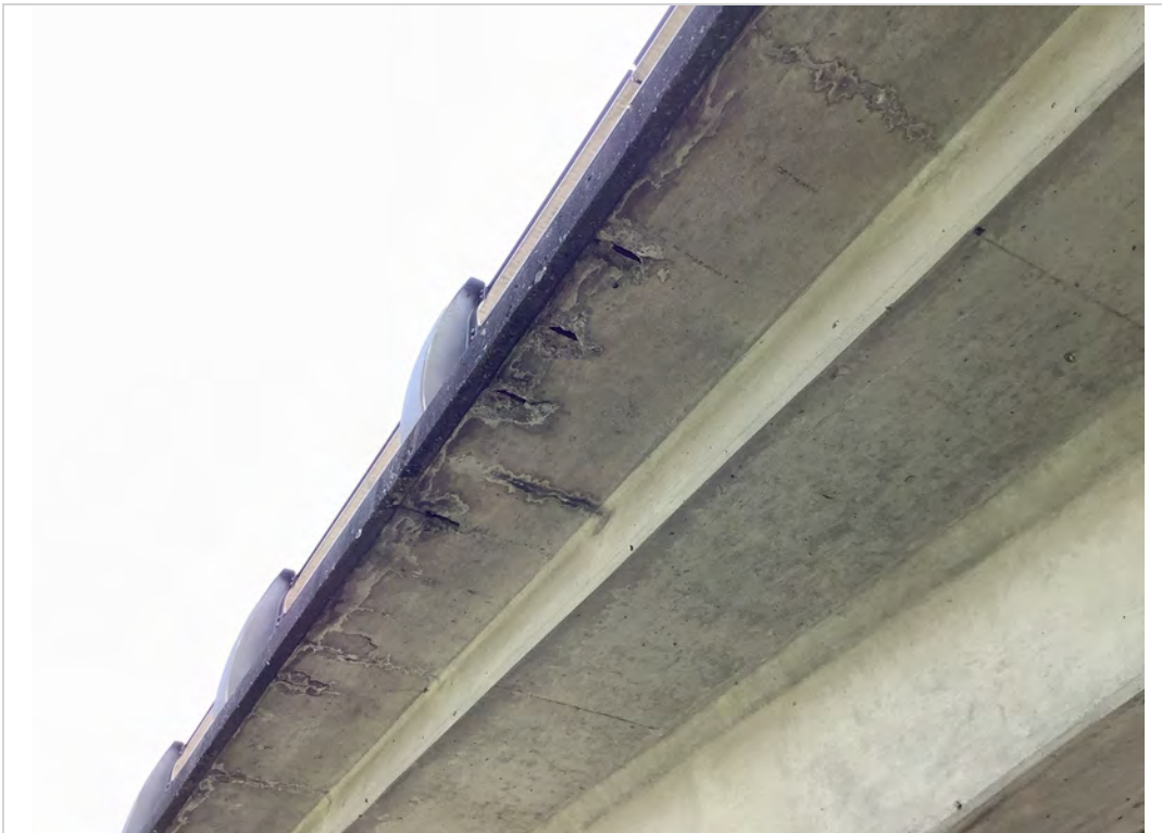
Typical spall with exposed rebar
